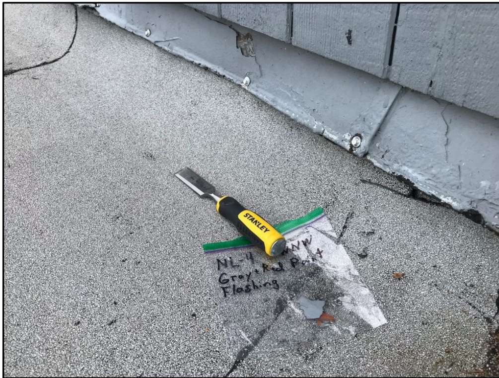
Sample – NL-4: NW Classroom Wing, WNW roof flashing: Gray & Red paint
